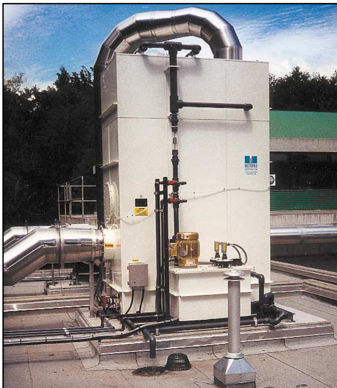
Duall PT-MD Packaged Wet Chemical Scrubber
